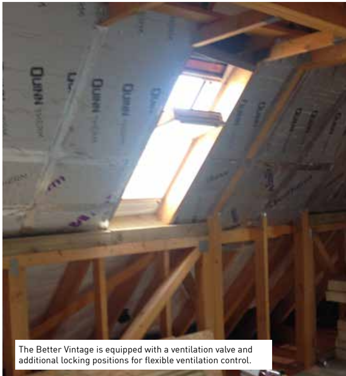
The underfelt foil collar included with the Better Vintage helps for a quick and easy installation
